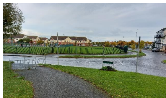
Image 2-3: No safe crossing provided on arm of roundabout.
